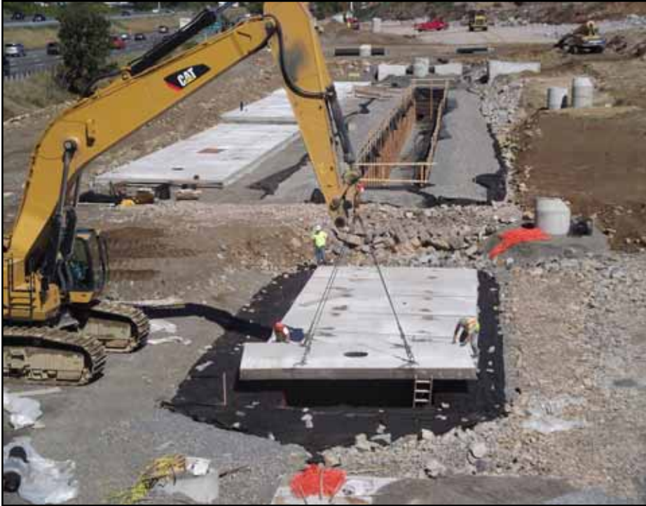
Roof slab installation.
