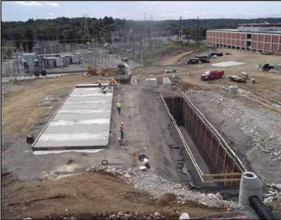
On-site construction of reinforced concrete roof panels.
