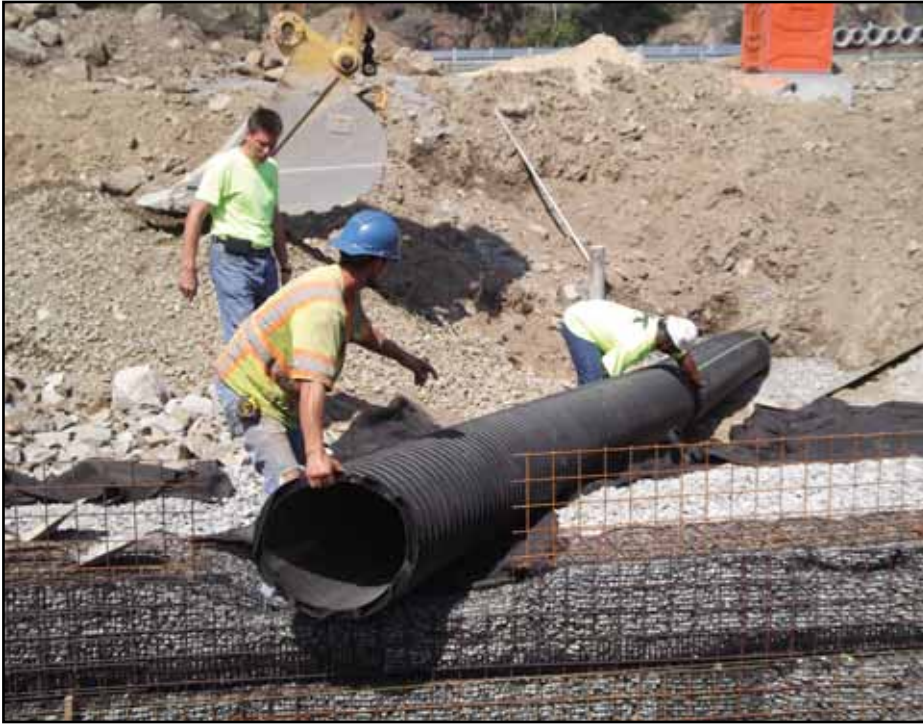
Inlet pipe installation.
