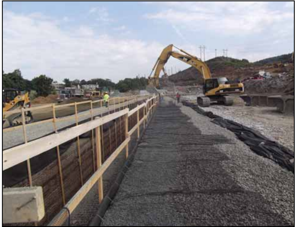
Chamber wall construction: stone backfill placed in lifts above geogrid reinforcement.
